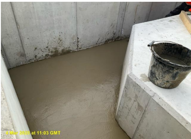
First pour to the chemical delivery bay
