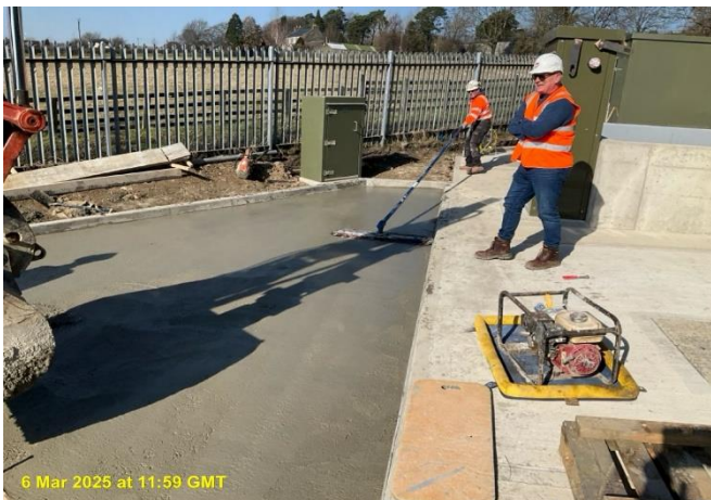
First pour to the chemical delivery bay
