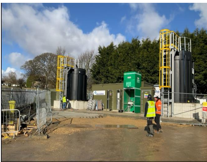
Commenced with the installation of the dosing equipment
