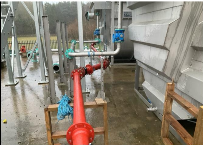
Pipe work fitted to the new unit
